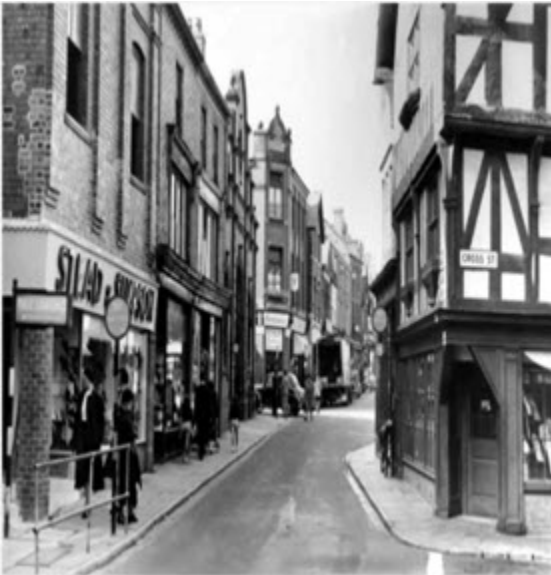
Bailey Street, Junction with Cross Street
